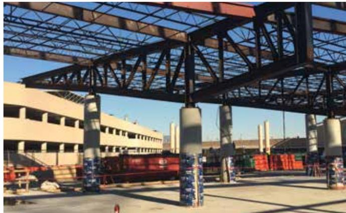
Figure 4. Cantilevered low roof truss supporting high roof framing.
