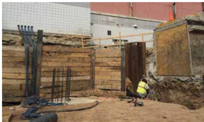
Figure 6. Soil retention system at existing electrical room.
